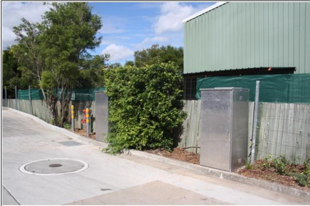
**Figure 5 - Sampler enclosures with treatment device in foreground**
